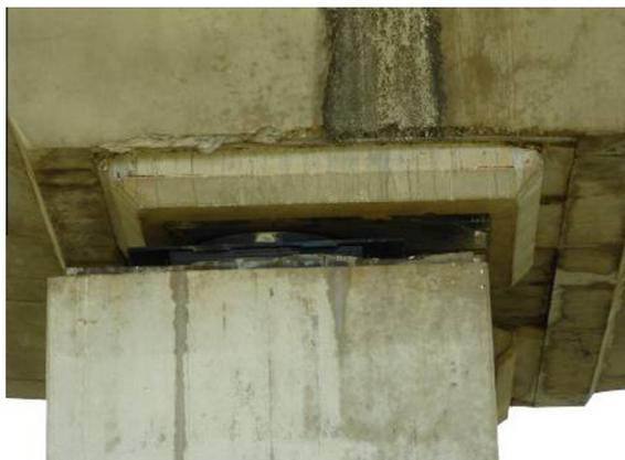
**Fig. 4.** Sliding displacement of a bearing device.
