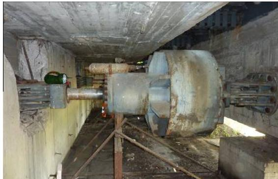
**Fig. 3.** Upstream abutments: dampers in extension.
