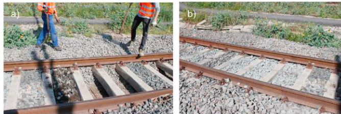
Fig. 2. (a) a set of three volumes emptied out of the original ballast; (b) the re-arranged configuration filled up with controlled material.
