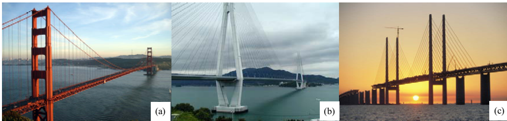
Fig. 2. (a) Golden Gate suspension Bridge (San Francisco, USA, 1937); (b) Tatarafan fan cable-stayed Bridge (Japan; 1999); (c) Øresund harp cable-stayed Bridge (Denmark, 2000)
