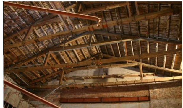
Fig. 32. The queen-post trusses of “Teatro Zandonai” (Rovereto, Italy) [38].
