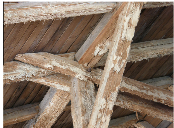
Fig. 4. Truss construction in the former brewery in Děčín.
