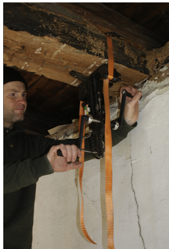
Fig. 26. Investigation of a tie beam condition using pin pushing.
