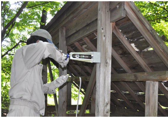
Fig. 42. Measurement of timber roof frames in Tsukuba City.
