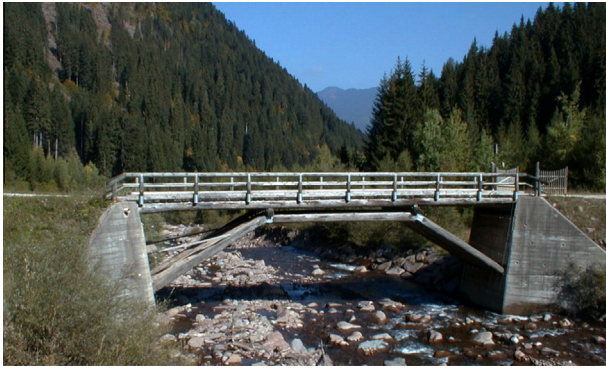
Fig. 33. Val Cadino timber bridge [39].
