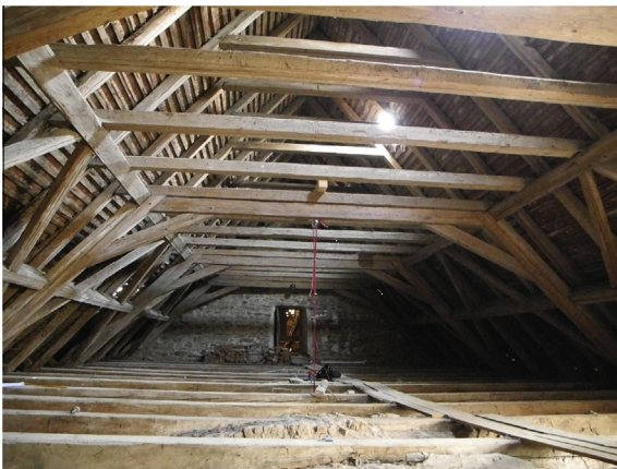
Fig. 19. Truss of the St. Mary's Church in Vranov nad Dyjí.
