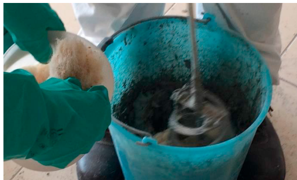
Fig. 5. Preparation of mortar.
