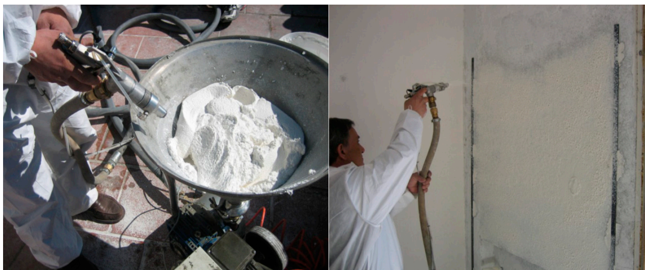
Figure 2. In situ application of the aerogel-based plaster.
