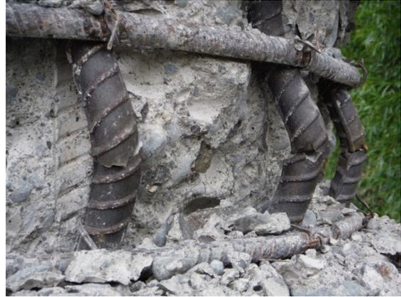
Figure 2 Fractured longitudinal reinforcing bars in a bridge pier close to the Mw 7.8 Kaikoura earthquake epicentre.
