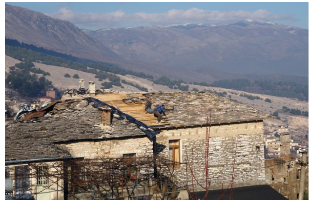
Figure 10. Traditional roof under restoration (© L.Dipasquale, 2019).
