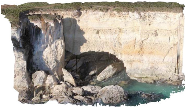
Figure 5: Orthophoto with an arched cavity
