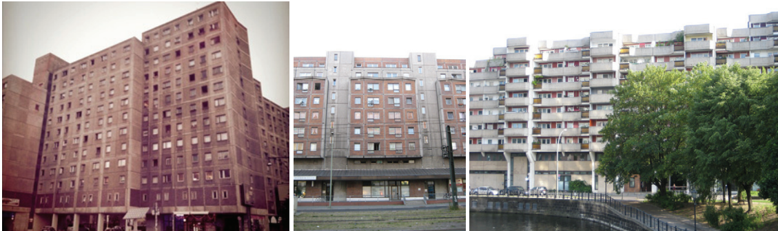
Fig. 1. (a); (b); (c) Residential building stock in Berlin: it needs strategy of social, morphological and re-use regeneration.
