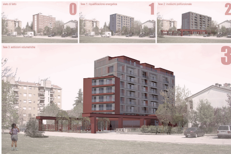
Fig. 3. Retrofitting of a social housing building in Forli, Emilia Romagna region. The building, which was erected during the '80s, has 8 floors and contains 34 flats. The project strategy provides these progressive stages: Phase 0, current situation: the overall energy performance index (Eptot) 153.37 kWh/m 2 y; Phase 1, retrofitting of the envelope: the overall energy performance index (Eptot) 55.98 kWh/m 2 y (63% decrease); Phase 2, integration of balconies, greenhouses and systems: the overall energy performance index (Eptot) 17.12 kWh/m 2 y (89% reduction); Phase 3, addition of high efficiency volumes: the overall energy performance index (Eptot) 13.40 kWh/m 2 y (91% reduction).
