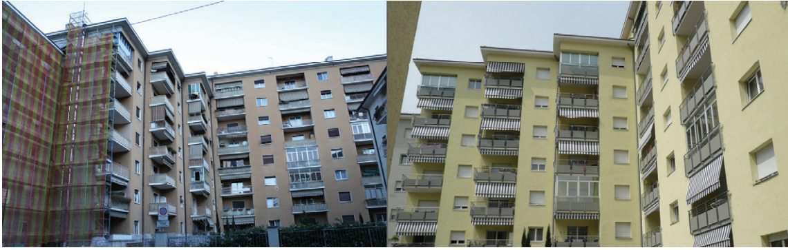
Fig. 2. (a) Regeneration of social housing complex in Bolzano (IT). The building, with 70 flats, was erected during '50s. The picture shows the building before the intervention; (b) The energy retrofitting of the envelope and the installation of centralized systems have improved the indoor comfort with an energy requirement of less than 40 kWh/m 2 y and a cost of intervention of 500 €/m 2 . The average cost for heating is 237 €. This is the first retrofitting intervention classified CasaClima B.
