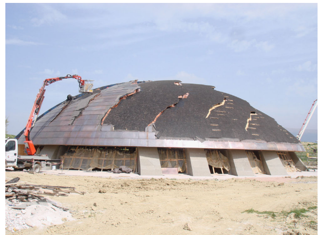
Figure 7 Placement of numerous copper plates on the roof.
