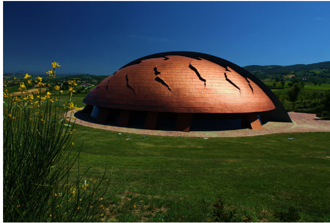
Figure 1 The Carapace at Castelbuono Estate Winery upon complete construction.
