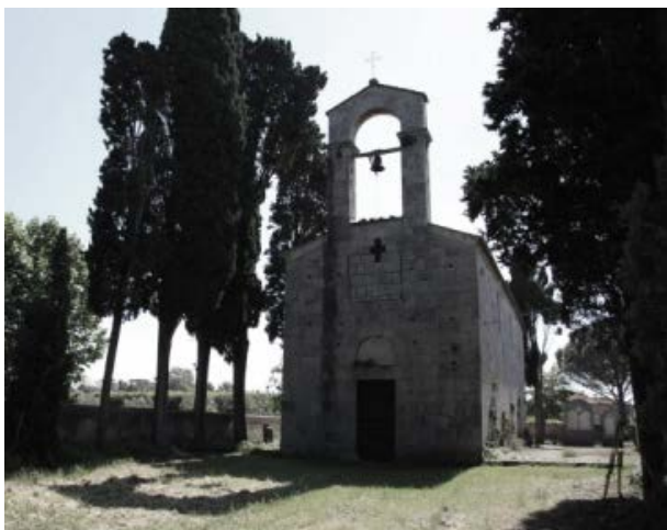
Figure 2. San Miniato church, the main façade
