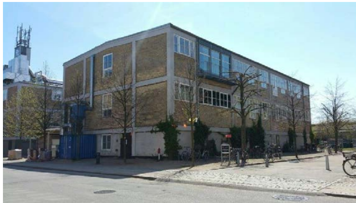
Fig. 1. Building 155- KADK Copenhagen
