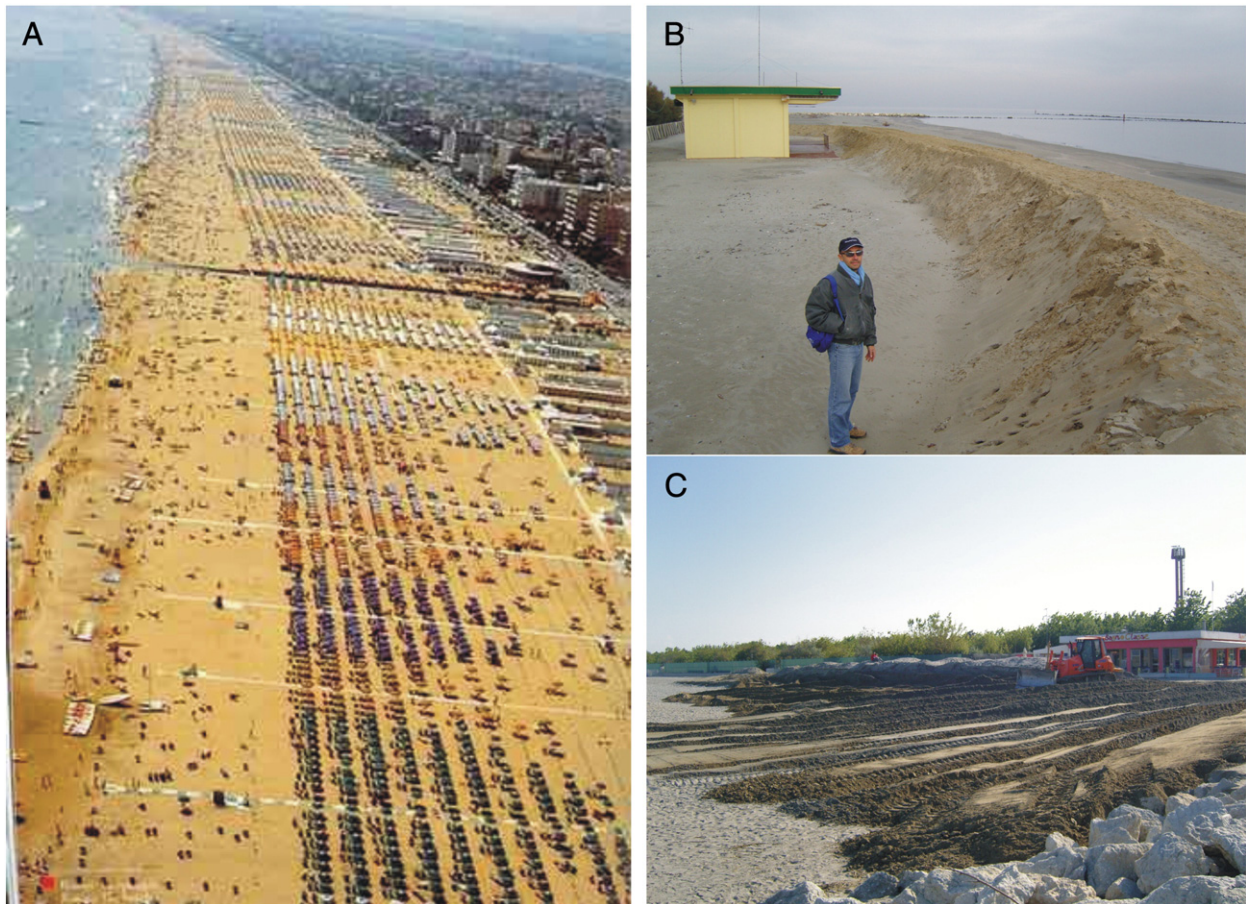
Fig. 1. (A) View of the beach in the Rimini area, Emilia Romagna Region. To note the intense urbanisation and occupation of the beach by tourist activities during the summer season (from the internet: http://xoomer.virgilio.it/hotel-rimini/Vacanze-Rimini-Riccione-Estate.jpg ); (B) example of artificial sand embankment built by beach users to serve as flood protection (November 2008); (C) the sand is bulldozed back to the lower beach at the beginning of the bathing season (May 2008). This creates unnatural beach slopes.
