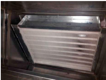
Figure 1. Coated Finned coil for heat and mass transfer
