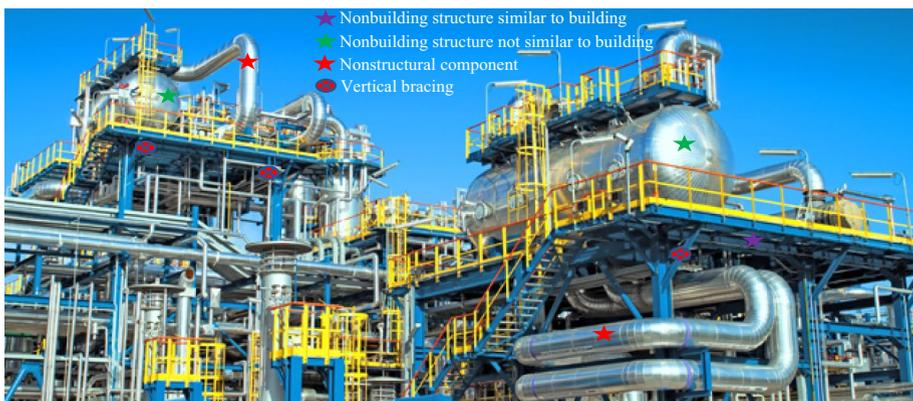
**Fig. 1** Typical configuration of nonstructural components and nonbuilding structures within a process plant (<http://www.pentechglobal.com/en>)
