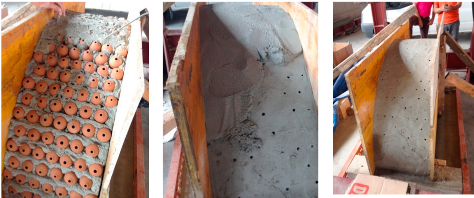
Fig. 2. Phase of realization of the masonry arch.
