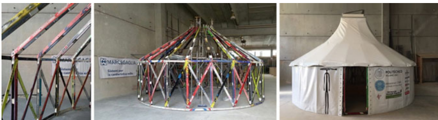
Fig. 8 Pictures of the pre-assembly phase
