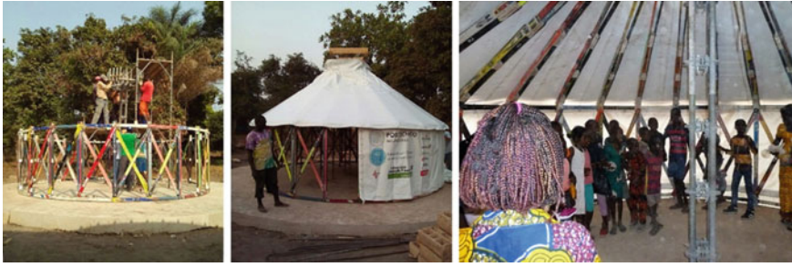
Fig. 11 Construction phases in Cacine, Guinea-Bissau
