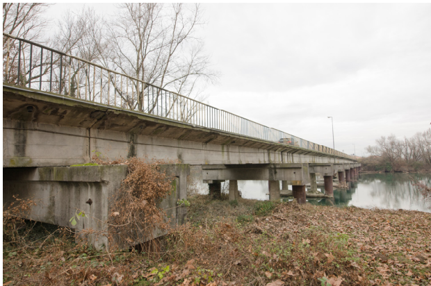
Figure 4. Current state of the bridge
