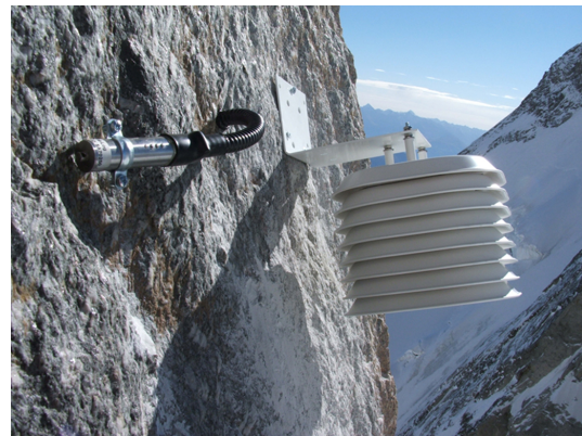
Fig. 5. The instruments installed on the near vertical rock-walls underlying the J. A. Carrel hut: in the foreground the mini-datalogger M-Log6 for the ground surface temperature measures and the radiation-shield hosting the M-Log5 for the measure of the air temperature.
