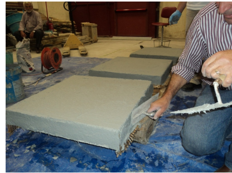
Figure 10: Drawing up of the second mortar layer 4 mm
