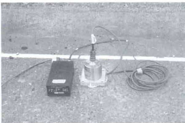
Fig.7 Installation of accelerometers on deck
