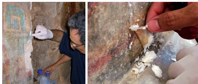
Fig. 5 The picture on the left illustrates the application procedure of the EAPC system. A cellulose poultice impregnated with EAPC is applied over the painting surface, previously protected with a Japanese paper tissue. On the right, the removal of the poultice after the cleaning procedure is shown.
