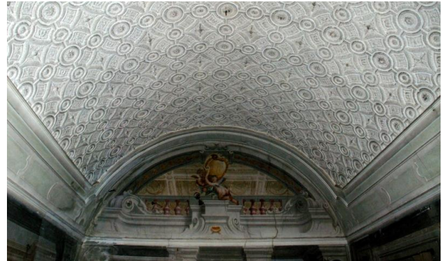
Figure 3. The vault of one minor room
