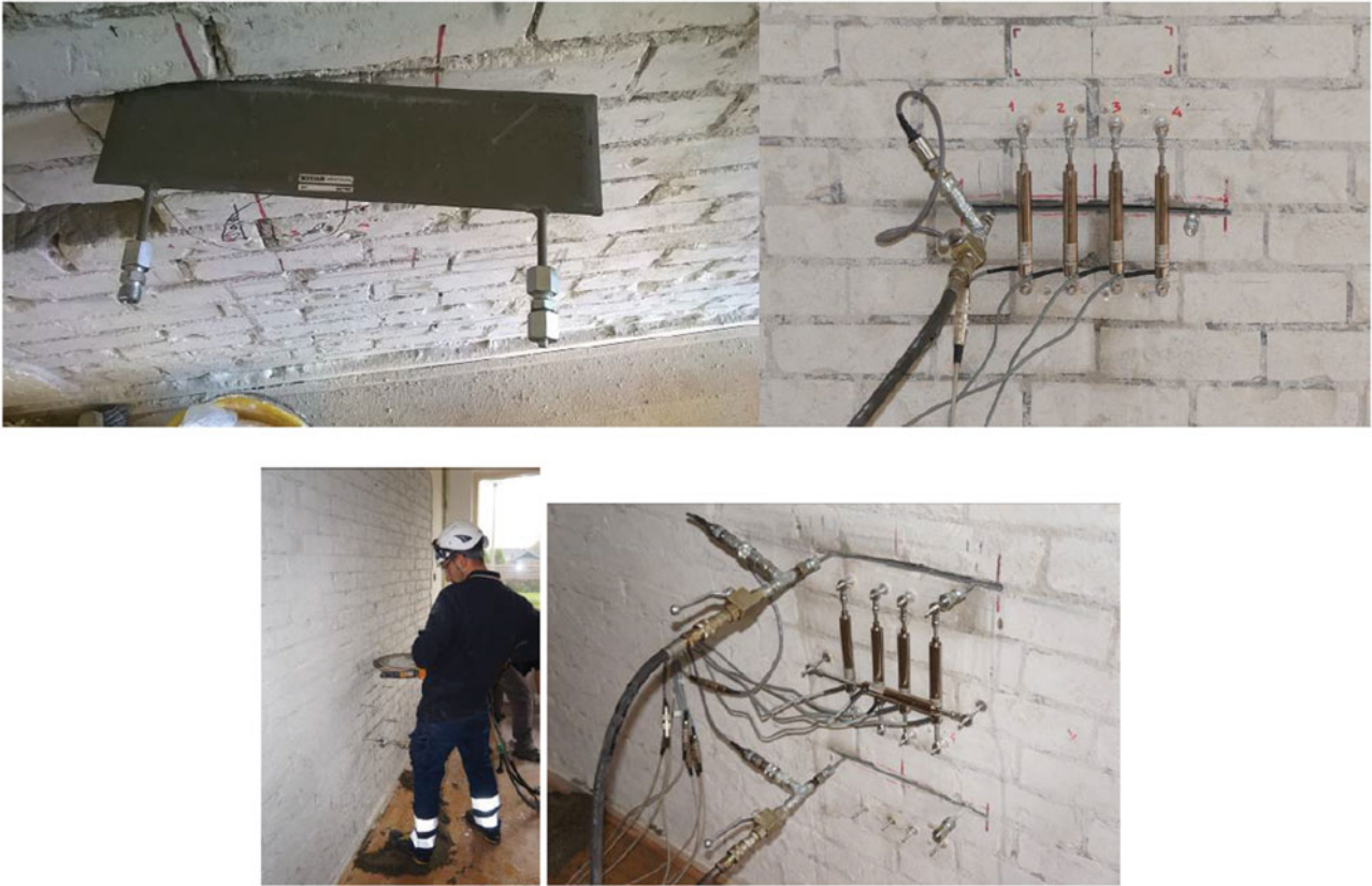
Fig. 3. In situ material tests on walls inside masonry houses (Eucentre et al., 2015).
