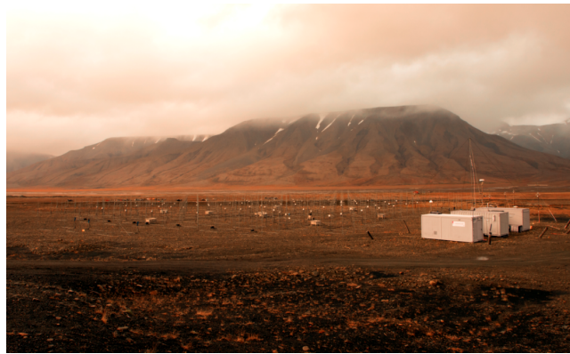
Figure 4. Sousy Radar Station in Adventdalen Valley 78^{\circ}10'10.05'' N, 15^{\circ}59'33.32'' E, Longyearbyen, Spitsbergen (Norway).
