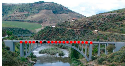
Fig. 1– Picture of the bridge taken from upstream, with the indication of the sections instrumented during the AVT (reference section in black).
