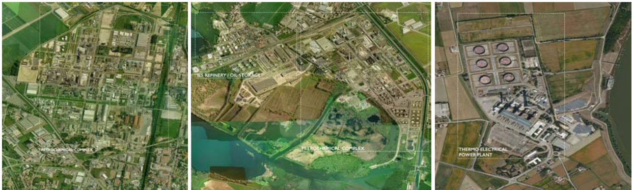
Fig. 6-7-8. Ferrara, Mantua and Sermide existing oil infrastructures.
