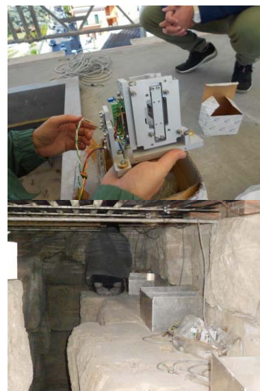
Figure 10. Installation of accelerometers, on the Attic of Trajan Arc
