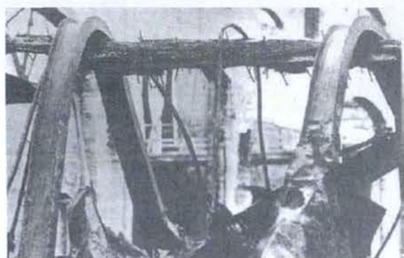
Fig. 12 Steel-timber structure in fire
