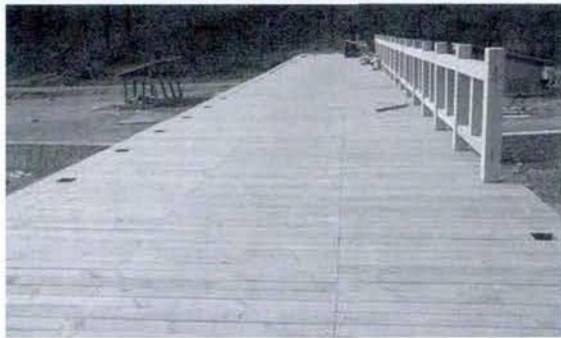
(b) Bridge under construction
