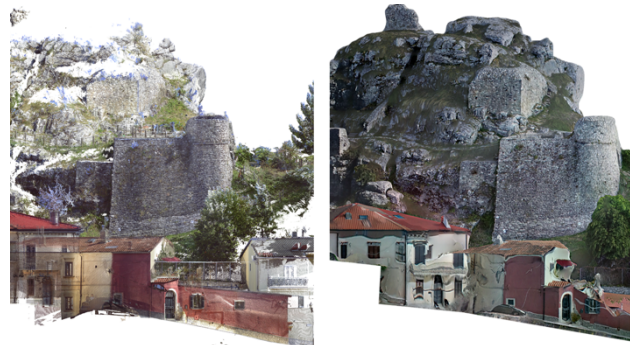
Figure 9. To the left: elevation of the Angevin tower in the laser scanner scans.
