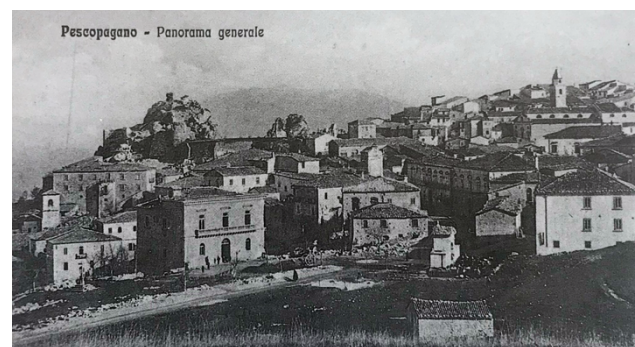
Figure 4. General panorama of the municipality of Pescopagano with the ruined castle. Date of the postmark: 19/08/1914 (Luccioni, 1988, p. 37).
