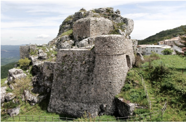
Figure 12. The Angevin tower (photo by UAV of 11/05/2019).
