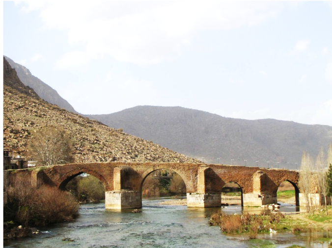
Fig. 1. Photograph of the Historic BISTOON Masonry Arch Bridge in Iran
