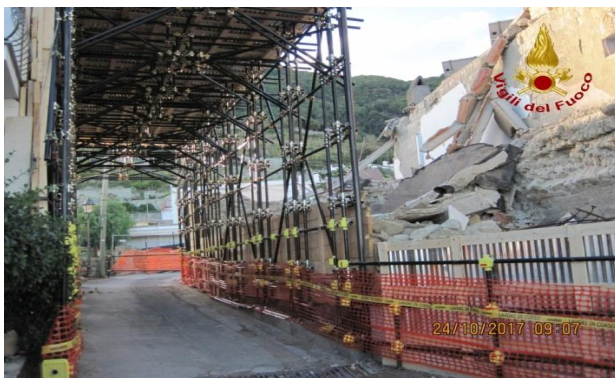
Figure 17. Tunnel with joint pipes
