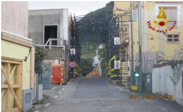
Figure 16. Bridge support structures
