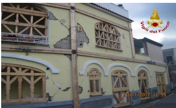
Figure 18. Examples of wooden planking for windows
