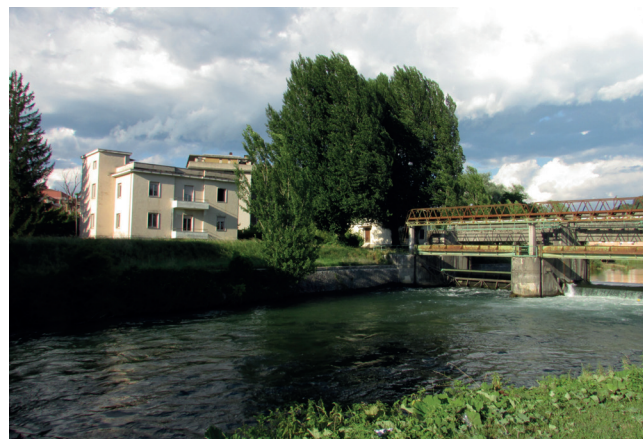
Fig. 5 - The barrage dam for water derivation and distribution at Voto dei Santi. The building at left (right bank of Velino River) is the Consortium for Rieti Land Reclamation headquarter (from Land Reclamation Authority collection).
