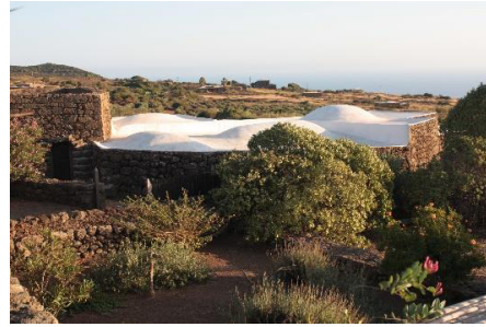
Fig. 6. Roof of Dammuso
