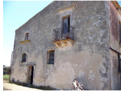
Fig. 4. Masseria with two-storey building
