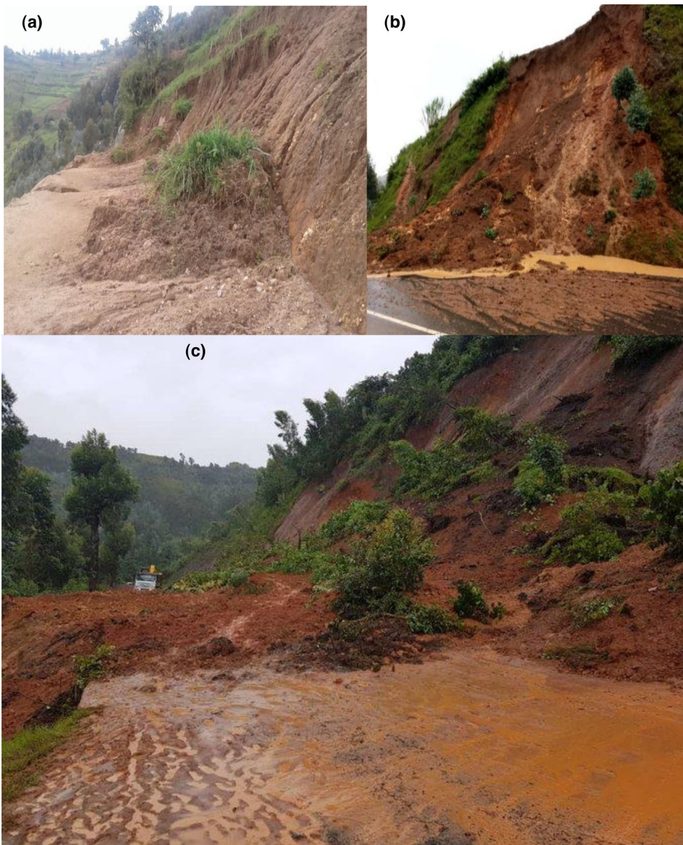
Figure 4. Fresh Landslide occurrences triggered by heavy rainfall in the study area (Source: Field visits by the researchers, June 2018-August 2019).
