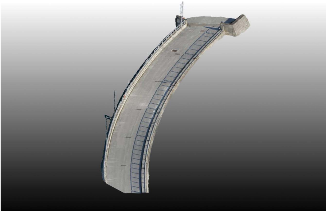
Figure 3. Texturized 3D mesh of the road way on the dam crest.
