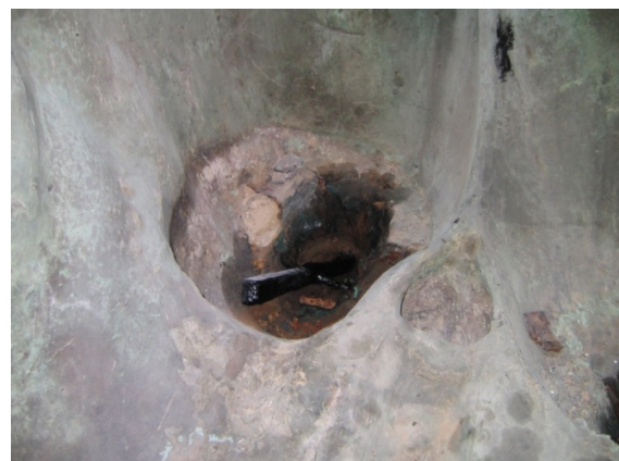
Figure 2: Detail of the internal part of the horse right foreleg showing the iron bar used as a reinforcement.
