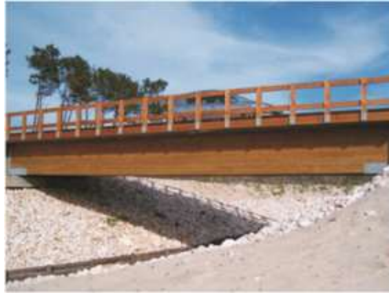
311 312 Fig. 19 TCC bridge after construction (courtesy of A.M.P.G. Dias).
