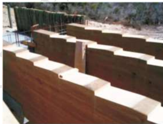
300 301 302 303 Fig. 15 Ends of glulam beams with triangular notches (courtesy of A.M.P.G. Dias).
