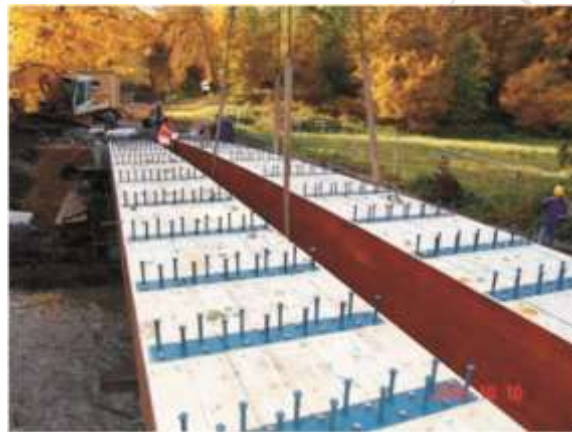
Fig. 21 Glulam sections with connectors before concrete placement (courtesy of P. Aldi).
