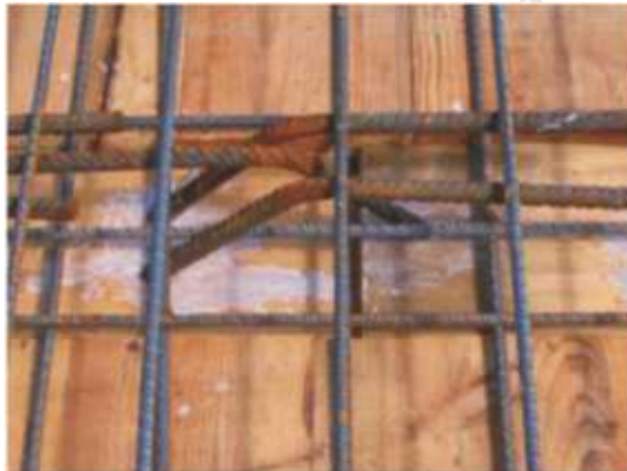
Fig. 17 Detail of the notch connection with inclined rebars (courtesy of A.M.P.G. Dias).
