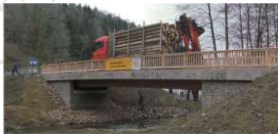
Fig. 22 TCC bridge built at Wippra, Germany, during the loading test (courtesy of P. Aldi).
