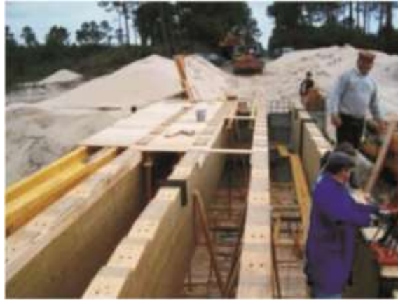
Fig. 16 Glulam beams with notches and holes for inclined rebars (courtesy of A.M.P.G. Dias).
