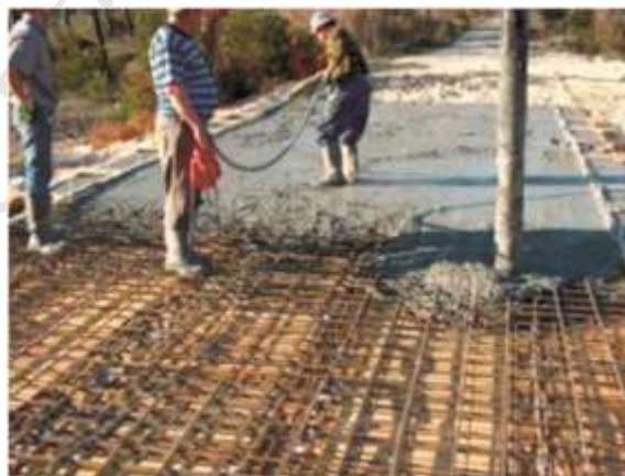
Fig. 18 Concrete placement (courtesy of A.M.P.G. Dias).
