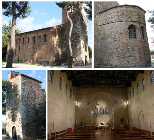
Figure 2. Photos of the outdoor and indoor of the church.
