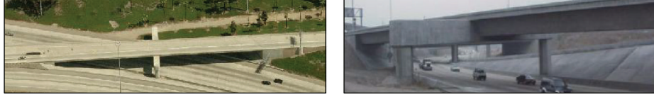
FIGURE 3: Two views of the benchmark highway bridge.
