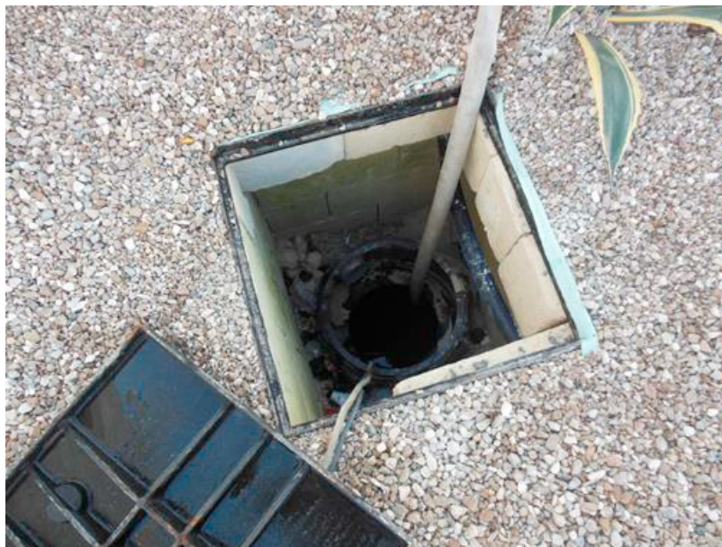
Figure 6 - Greywater tank.
