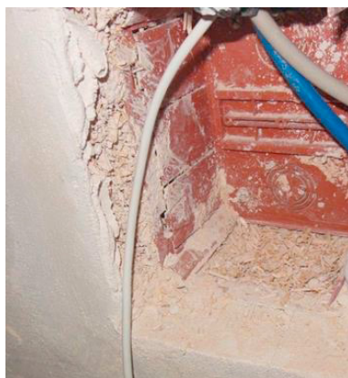
Figure 3 - Detail of Hemp-lime internal coat.
