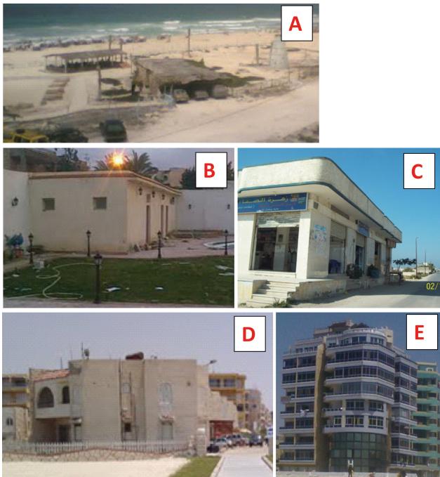
Figure 21. Typical constructions of classes from A to E in Alexandria (pictures from Google Earth database).
