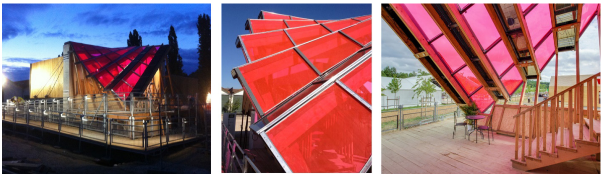
Fig.2. (a) Night view of the Liv-lib' during the SDE 2014 competition, showing; (b) The LSC panels stand out on the roof; (c) Under the canopy the light gets a red hue caused by the re-emitted light that doesn't undergo total internal reflection
