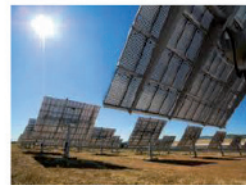
Fig. 6. – CPV is an opportunity to exploit the high triple-junction conversion efficiency.
