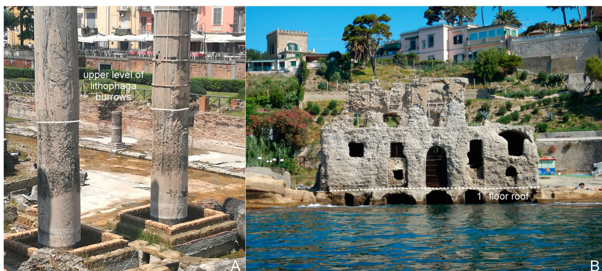
Figure 5. Evidence of post-Roman subsidence along the coast of Pozzuoli and Posillipo. A) Macellum columns with Lithophaga burrows up to 7 m a.s.l.; B) the Palazzo degli Spiriti Roman building with the first floor completely submerged.
