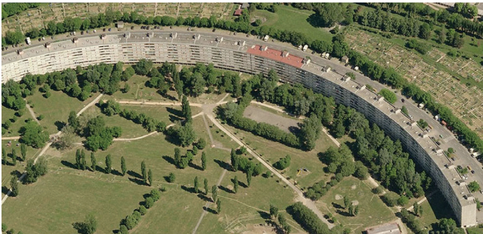
Fig. 3. Aerial view of the 700 meters long building named "Virgolone", built in 1975
