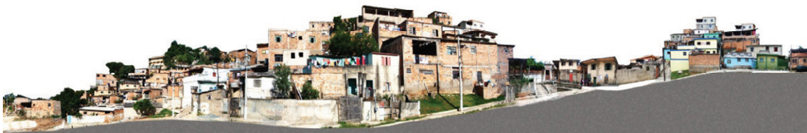
Fig. 3: The skyline from the main street “beco um” show the principal building materials employed.
