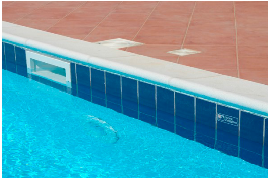
Figure 9 A detail of the pool with skimmer
