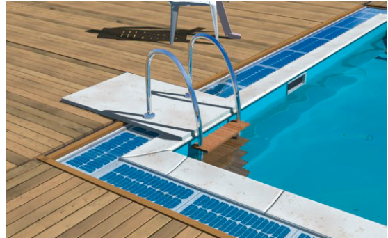
Figure 10 Outline of the edge for a skimmer pool
