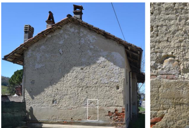
Figure 2. Earth plasters on adobe walls, Photo by the authors.
